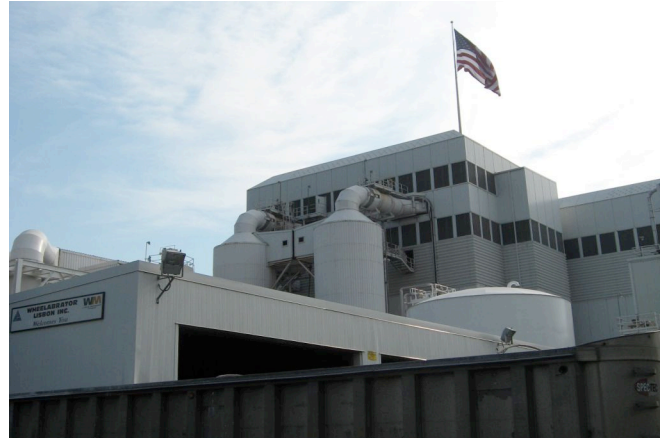
Lisbon, CT Waste to Energy Facility
