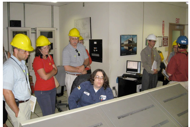
Wheelabrator Operator explains Pollution Control Monitoring
