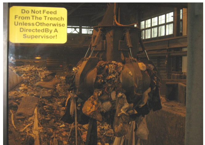
Over one ton of trash is grappled in each crane lift
