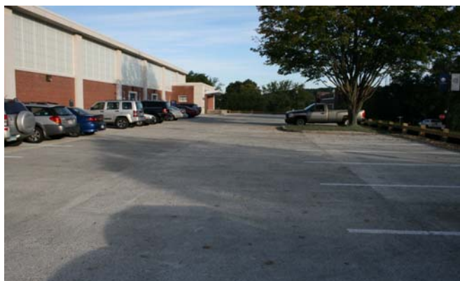
Completed Field House Parking Lot
