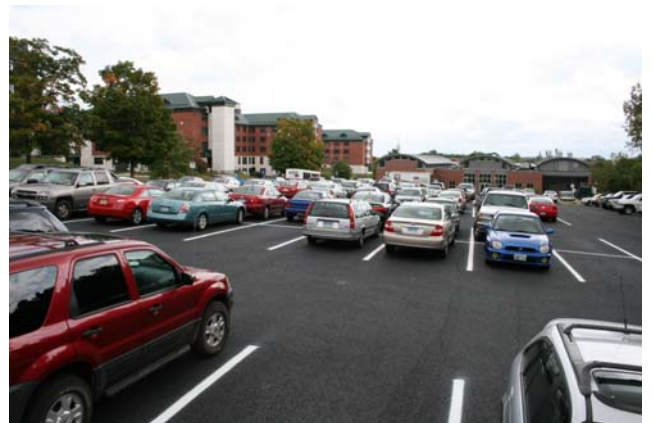
Completed Towers Parking Lot
