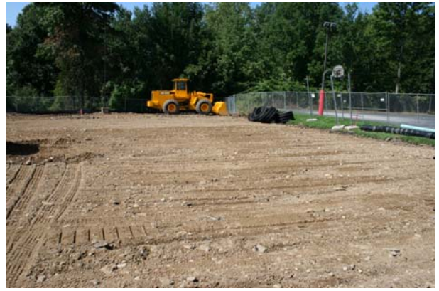
Removal of Towers Parking Lot
