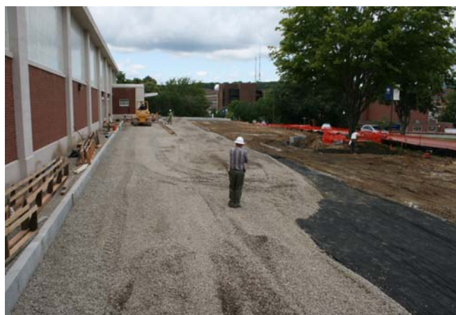
At Field House 6" of Pervious Concrete over 12" of Washed Stone
