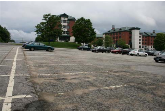
Prior Conditions at Towers Parking
