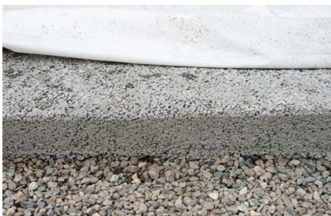
Field House Parking Lot Preparation for Improvements
