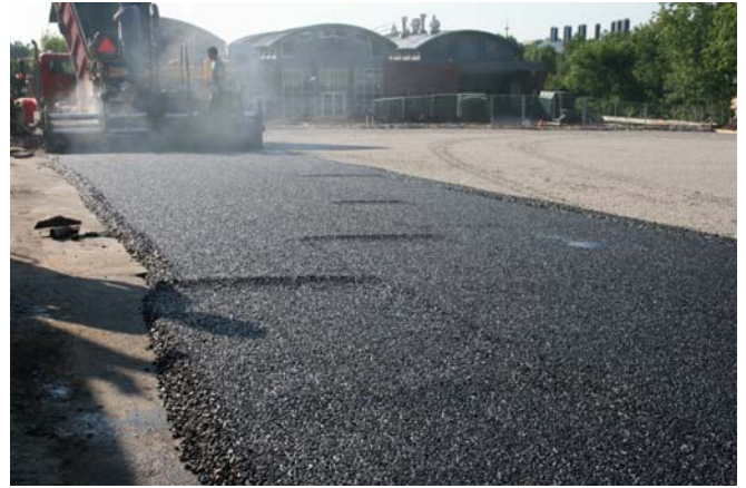
Pervious Pavement Installation at Towers Parking Lot
