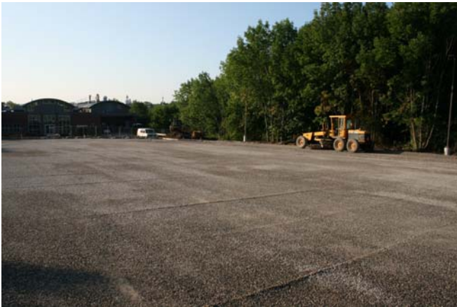
Choker Course Ready for Paving at Towers Parking Lot
