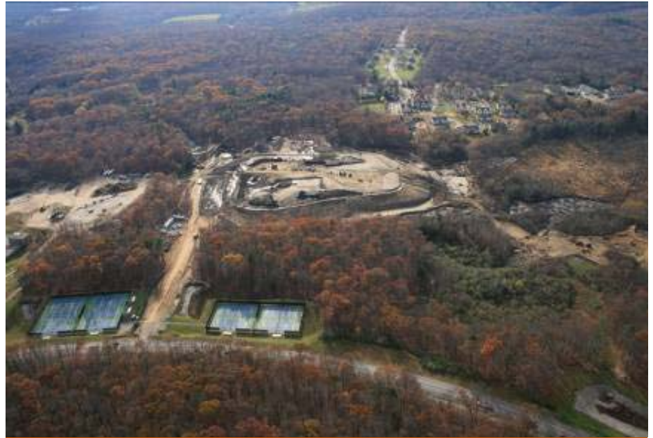
Aerial view of the remediation at the former UCONN landfill site.
